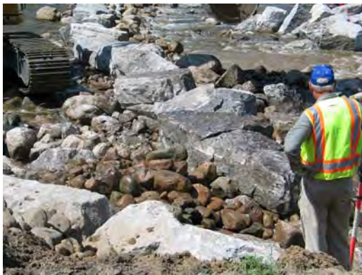
Working on the Chesaning Dam
