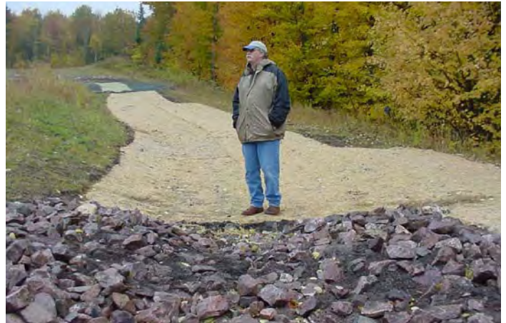
Alger Conservation District board member, Hampton Waring, inspects site following remediation
